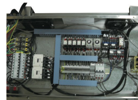
Spacy top-mounted electrical panel for easy service and maintenance.
